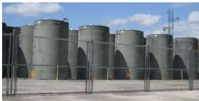
Figure 1.13. Dry cask storage of spent nuclear fuel at Vermont Yankee nuclear power plant [15].
